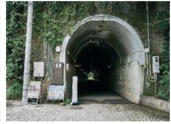
Tunnel at the start of the trail
