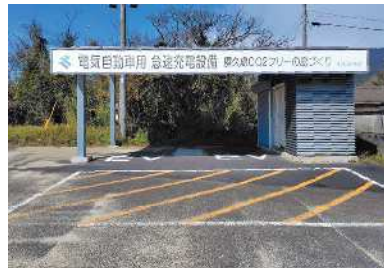
Rapid Charging Station
